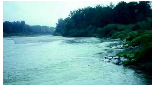
Figure 43: Field installation of stream barbs (USDA, 1996).
