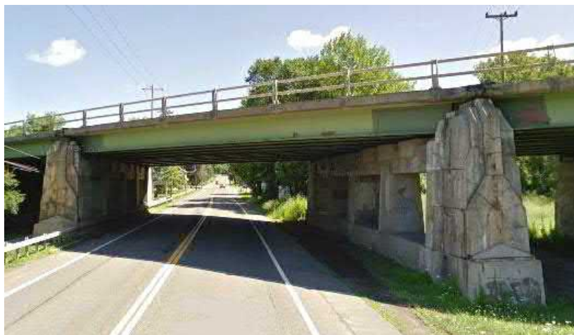
Figure 22 Existing conditions of the Route 9H Overpass, entering Valatie, NY
