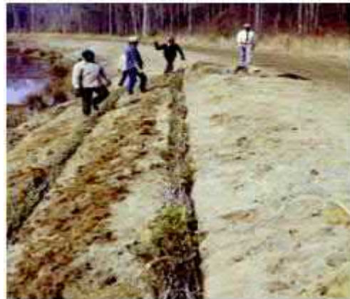
Figure 34: Live fascine slope stabilization (Photo courtesy USDA - Robbin B. Sotir & Associates).
